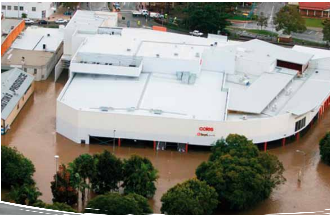
A commercial centre floods in 2009.
